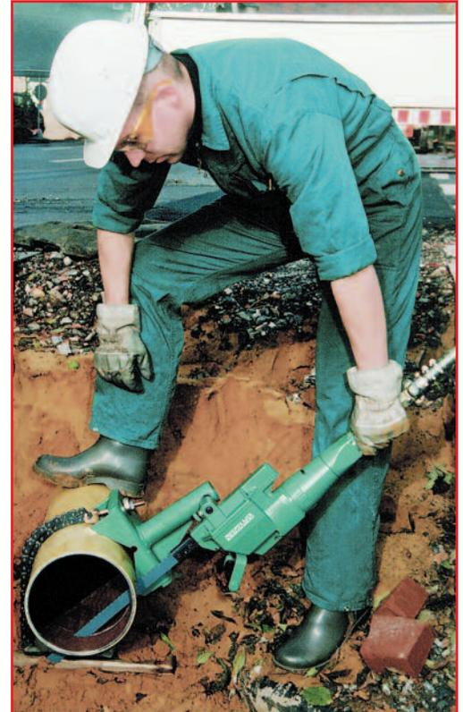
**Assorted pipe clamps for pipes up to 30" OD or profile clamps for structural steel (see pages 17-18)**
